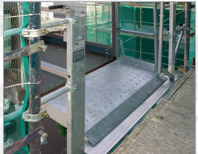
Landing with opened platform ramp
